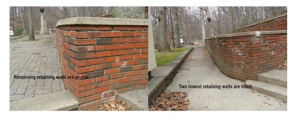
c. The walls are topped with **concrete** coping, rather than the described *stone*. A wash could be used to visually improve the look of unsightly existing repairs. Several sections require a new **concrete** cap.
