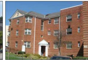
Lee Gardens North (Woodbury Park)
