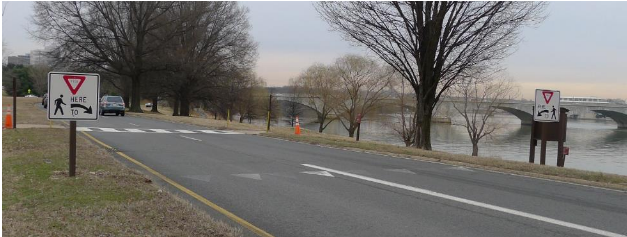
Example of pavement markings aligned with yield signs
